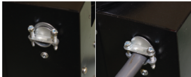
Figure 9: Installing cable fitting to heater
